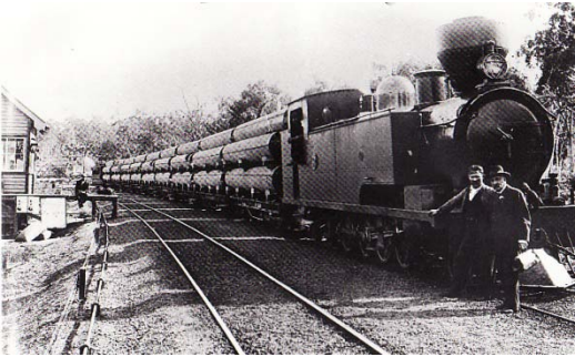
Train load pipes-ex Maylands c1900
